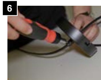
After adjusting cord length, tighten set screw on canopy.
